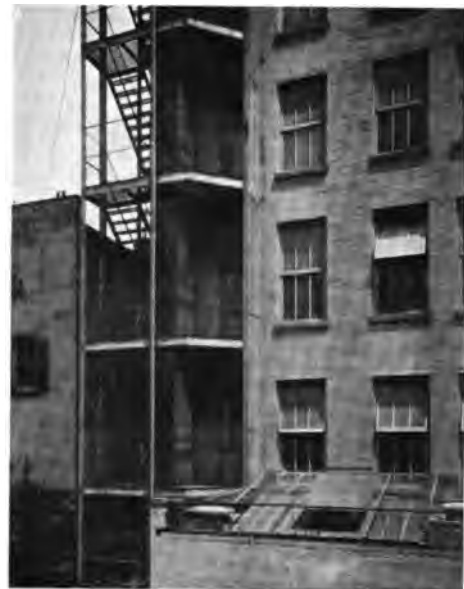
Fig. 2. Outside Stairway protected by Wing-Wall.*
